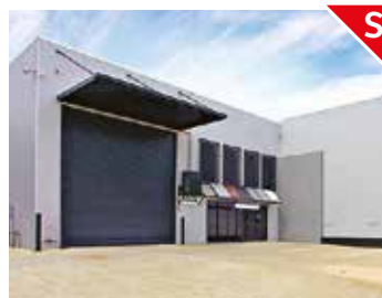
1/65-67 Steel Street, Capalaba Price: Sold $915,000 Building: 494 sqm Office: Bayside
