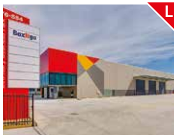
576 Boundary Road, Archerfield Leased: $1,152,363 pa (Net) Building: 1,178 - 2,080 sqm Office: Brisbane Southside
