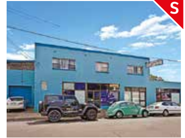
27-31 Milton Street North, Ashfield Sale Price: Price on application Land: 1,028 sqm Office: South Sydney
