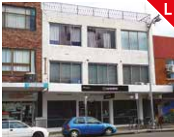
314-316 Marrickville Road, Marrickville Rent: $143,000 pa Building: 330 sqm Office: South Sydney
